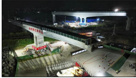
Figure 6.7 - Rotated bridge in Hubei
