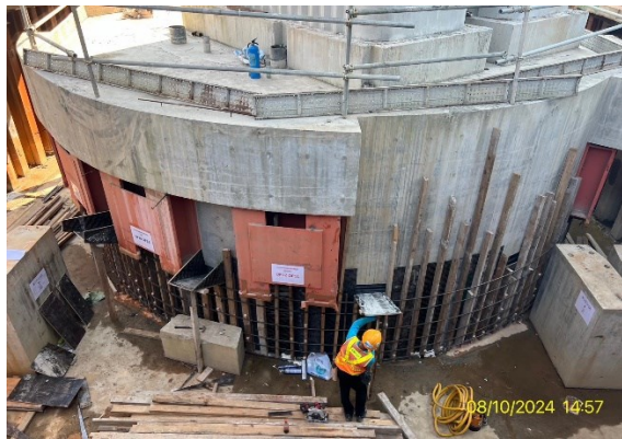
Figure 4.55 - Concreting for Stitch
