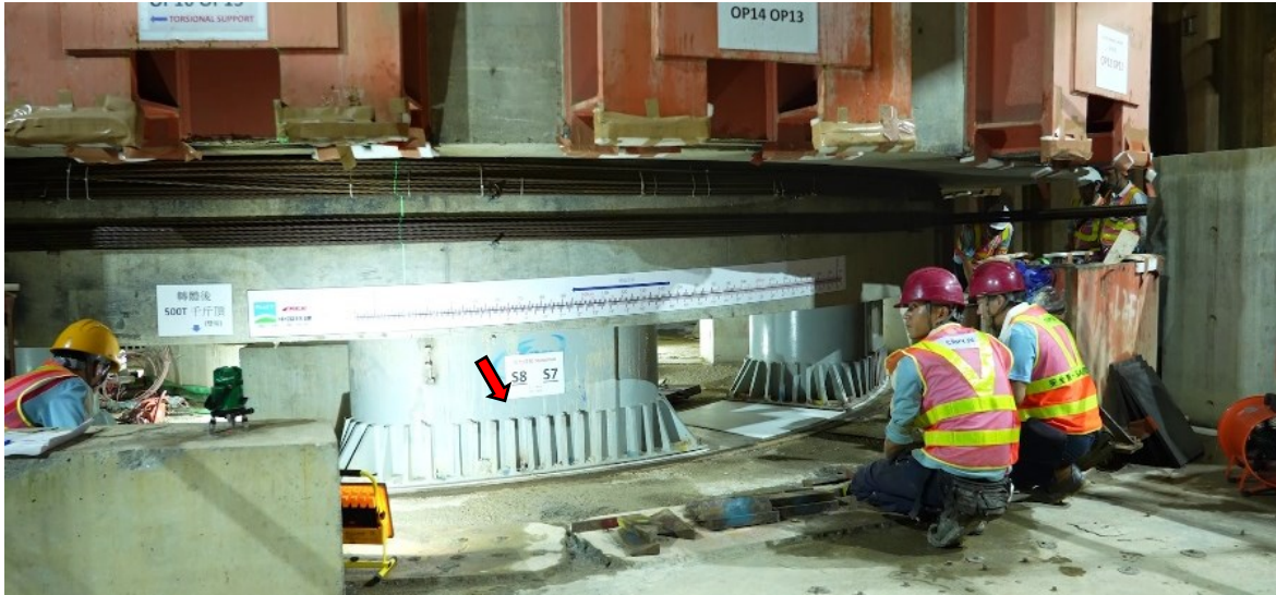
Figure 4.15 - Stanchions before rotation
