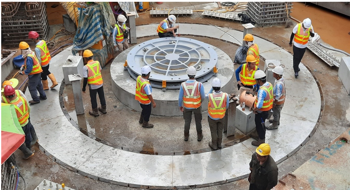
Figure 4.6 - Spherical Bearing Installation
