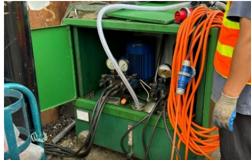
Figure 4.40 - Hydraulic pump for strand jack
