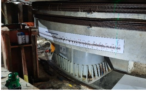
Figure 4.37 - PTFE sliding plate and the horizontal laser marker
