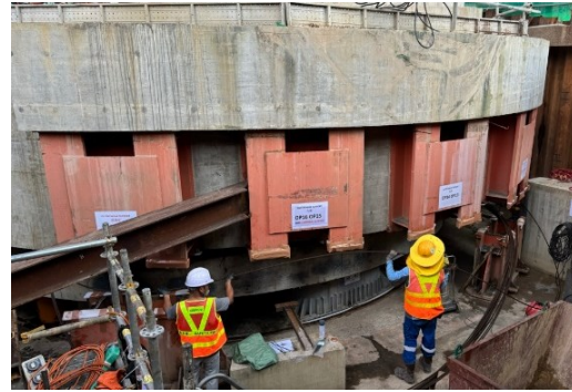
Figure 4.44 - Fixing traction strands
