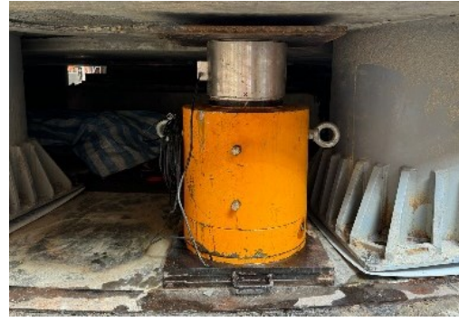
Figure 4.32 - Load cell on the hydraulic jacks
