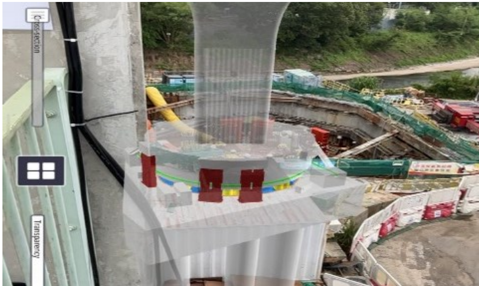
Figure 6.15 - Capture of Bridge Rotation Elements in the AR BIM Visualization
