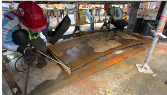
Figure 4.24 - Shimming and Spot Welding at Stanchion
