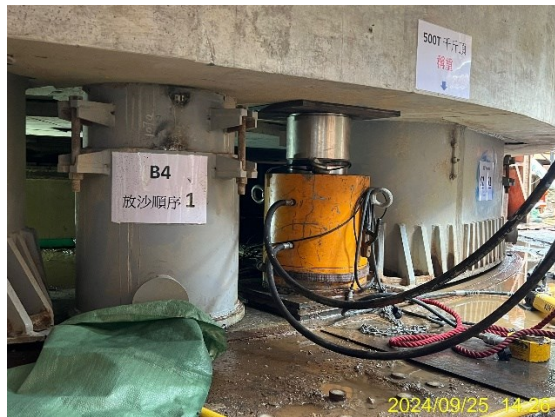
Figure 4.46 - Sandboxes and hydraulic jacks
