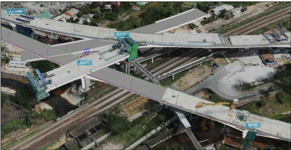
Figure 6.11 - Existing Conditions Modeling by Photogrammetry
