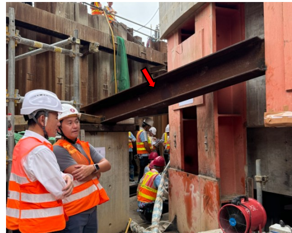
Figure 4.14 - Torsional support installed on upper turntable prior to removal of sandboxes
