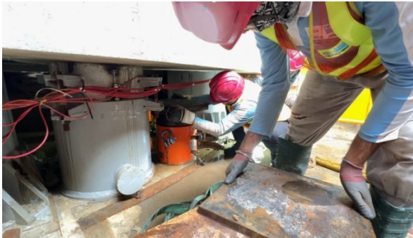
Figure 4.23 - 500 Ton Jack Installation
