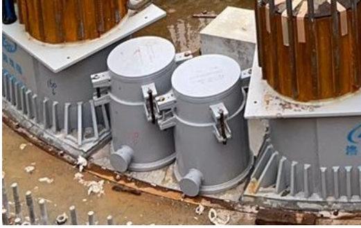
Figure 4.18 - Pre-load of the sandbox
