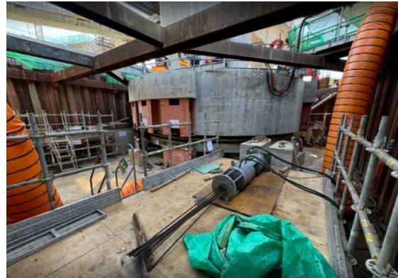
Figure 4.12 - Set-up of continuous strand jack at the primary reaction block
