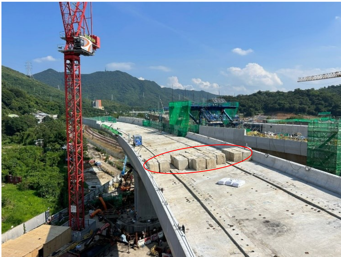
Figure 4.49 - Counterweight Concrete Blocks for Weight Balancing
