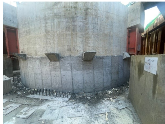
Figure 4.56 - Post-concreting condition of the stitch
