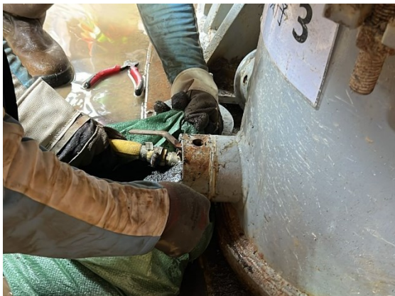
Figure 4.45 - Removing the quartz sand
