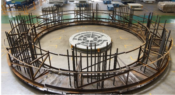
Figure 4.8 - Preassembled framework
