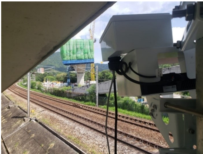
Figure 5.3 - LiDAR device along the railway track
