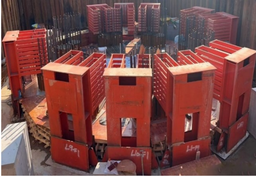
Figure 4.21 - Photos of turntable showing the inner and outer shear support
