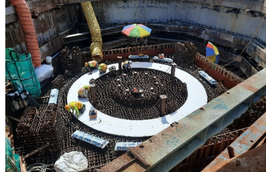
Figure 4.9 - Installation of sliding track
