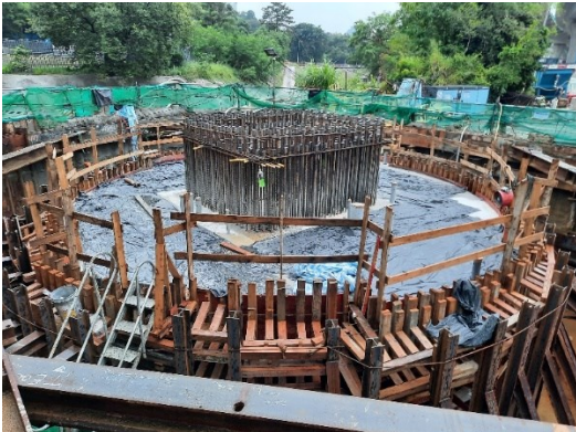
Figure 4.11 - Upper turntable casting
