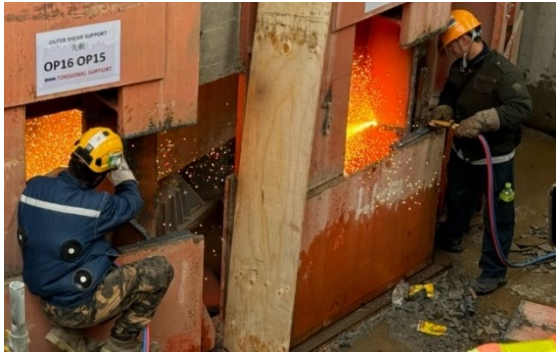
Figure 4.43 - Cutting of shear supports
